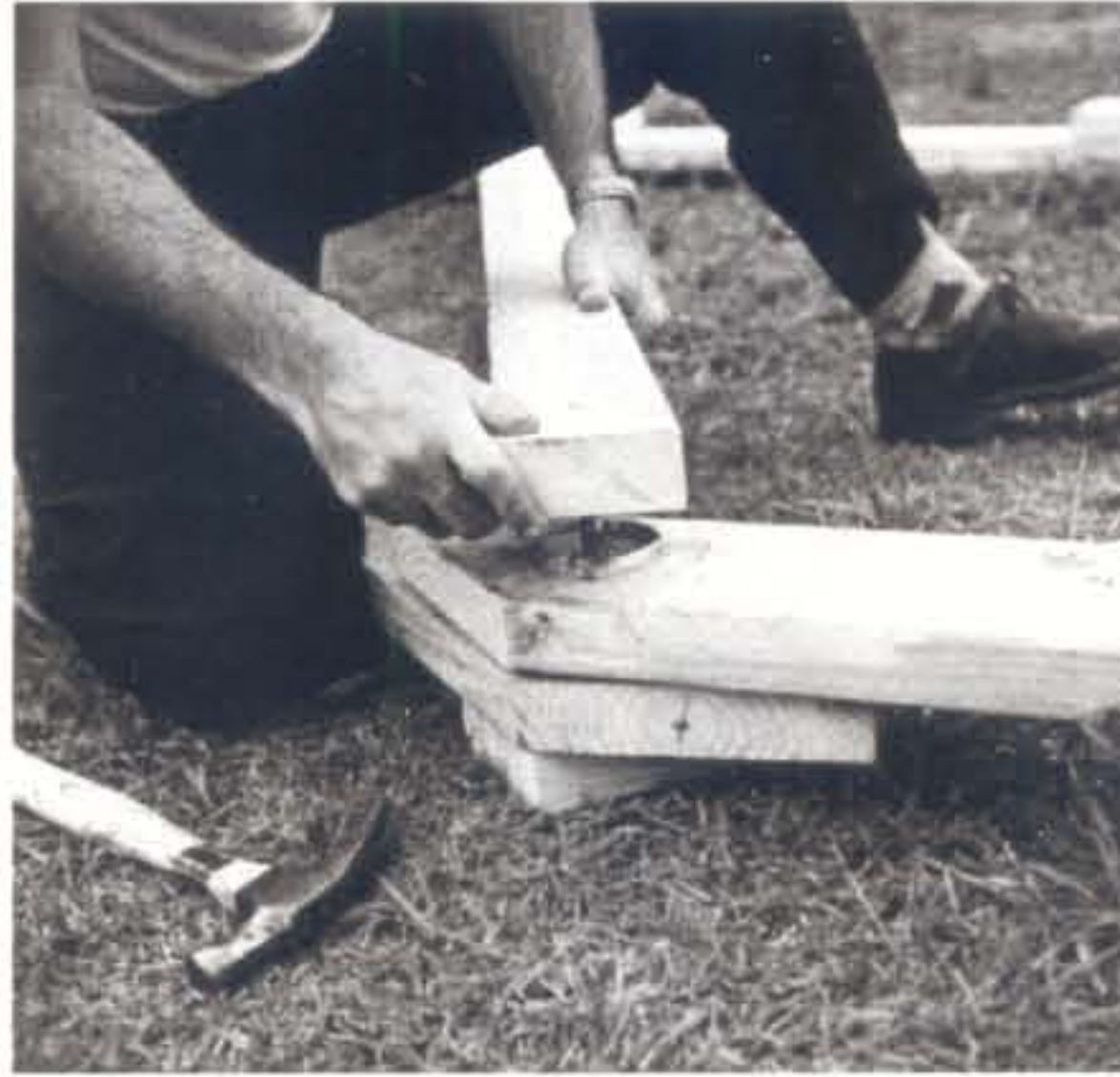
Assembling a timber joint with a TECO Wedge-Fit split-ring connector
