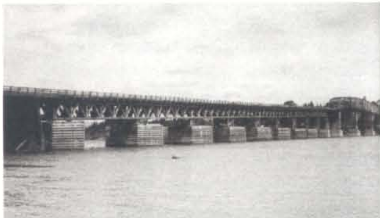
Wooden bridge over half of the Columbia River near Cathlamet, Washington. A 2,433-foot-long bridge built in 1938-39 and opened in 1939, used over 24,000 TECO split-ring connectors
